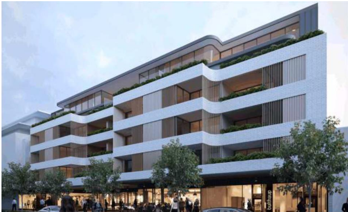
Figure 8 – Hunters Lodge (16-18 Cross Street ) Source: Bates Smart
